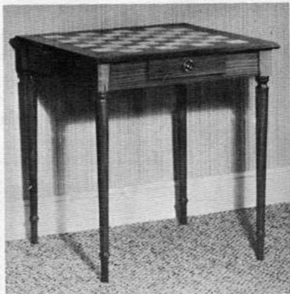
No. 765D CHESS TABLE. Large card table size 30" x 30" x 28" high made of solid walnut with white birch and walnut squares. Large drawer for Chess set. Turned legs screw into table top frame. Shipped with legs off. 2 1/4" squares. Packing 1 — 35 lbs.
